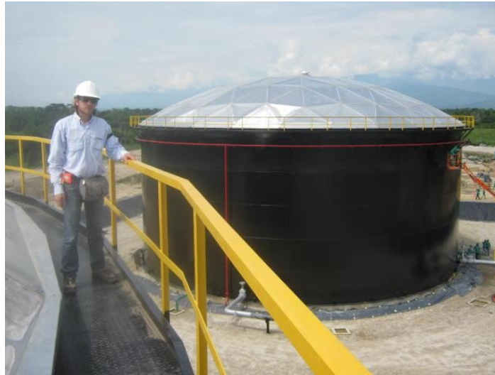
Tanque TK 4150 50 KBL-Banadia- Arauca2 Ecopetrol Colombia
